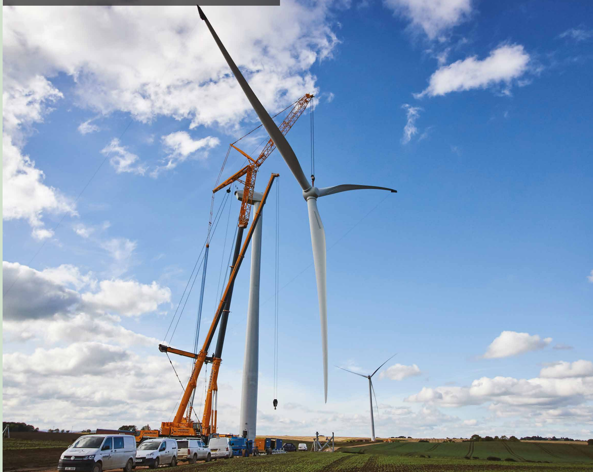
Turbine blade lift at Moor House Wind Farm
