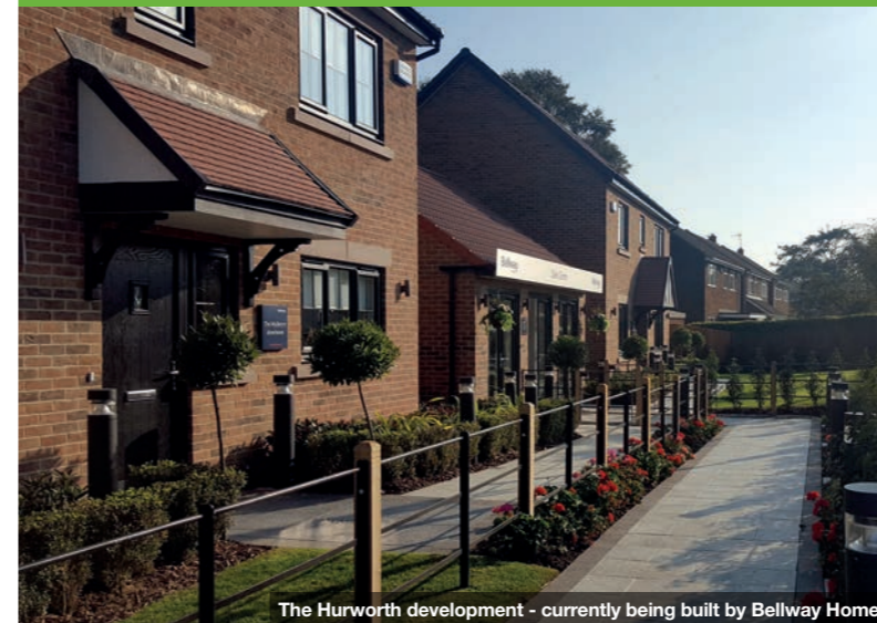
The Hurworth development - currently being built by Bellway Homes
