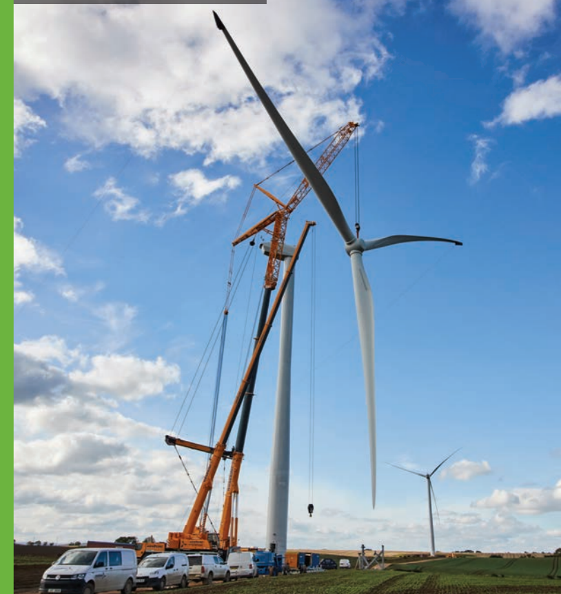
Turbine blade lift at Moor House Wind Farm
